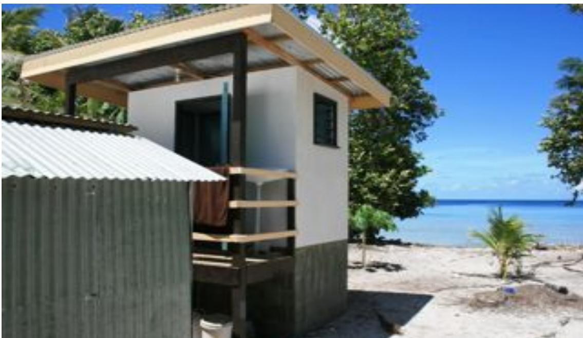
Figure 11: Composting toilet installed by the project. Prior to the installation of these toilets, waste seeped into groundwater and discharged into the lagoon
