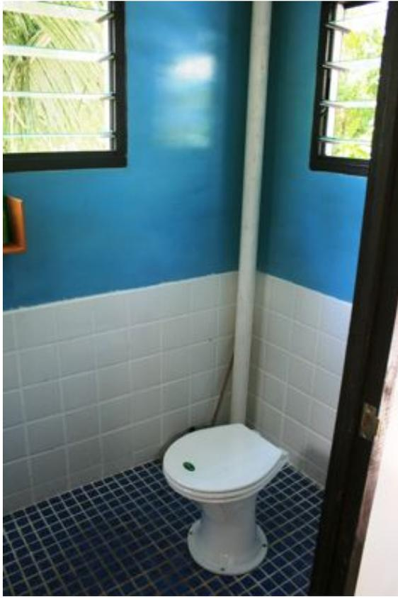
**Figure 12:** Waterless ecosanitation toilet installed by the project
