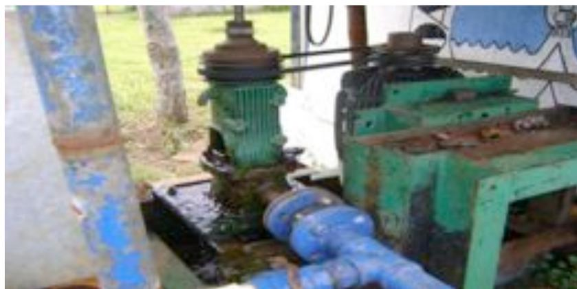
**Figure 19** Old infrastructure associated with 70% leakage losses. A key study suggest that old valves may be contributing significantly to losses
