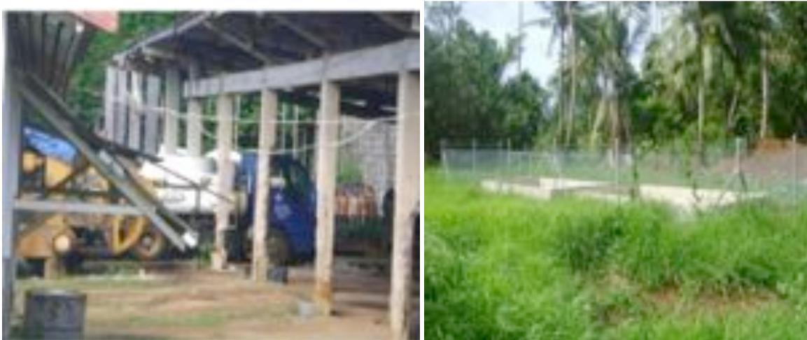
**Figures 17 & 18:** Vacuum truck and sludge management beds at Kalaka Site
