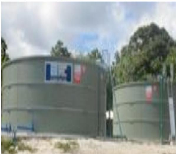
**Figure 9:** The two new 240 kL storage facilities at Alofi South
