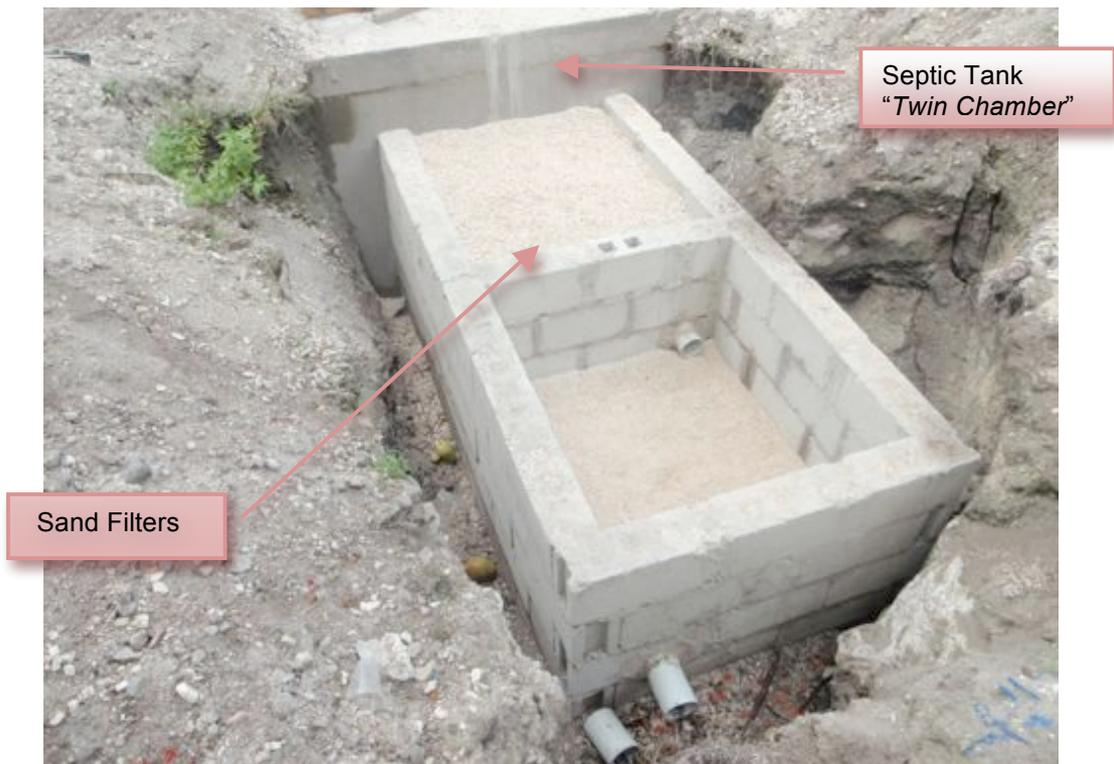
**Figure 7** Prototype #1: A Conventional Septic Tank “Twin Chamber” added with two stages Sand Filters as Secondary Treatment to improve the waste water effluent prior being discharge via irrigation.
