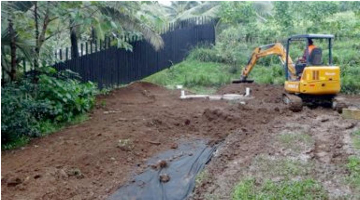
*Package secondary treatment plant and land application system being installed at homes in the Muri-Avana area*
