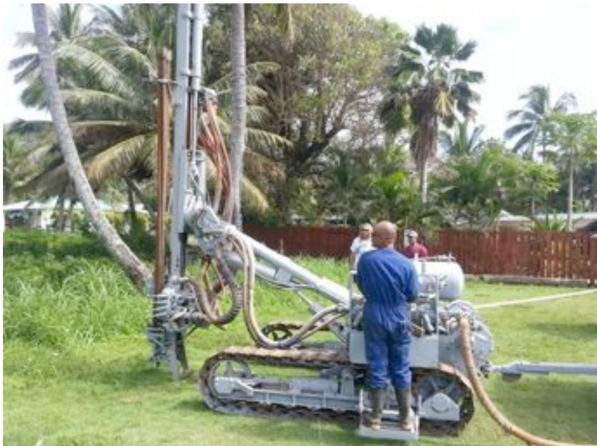
*Drilling groundwater monitoring wells in the demonstration project area*
