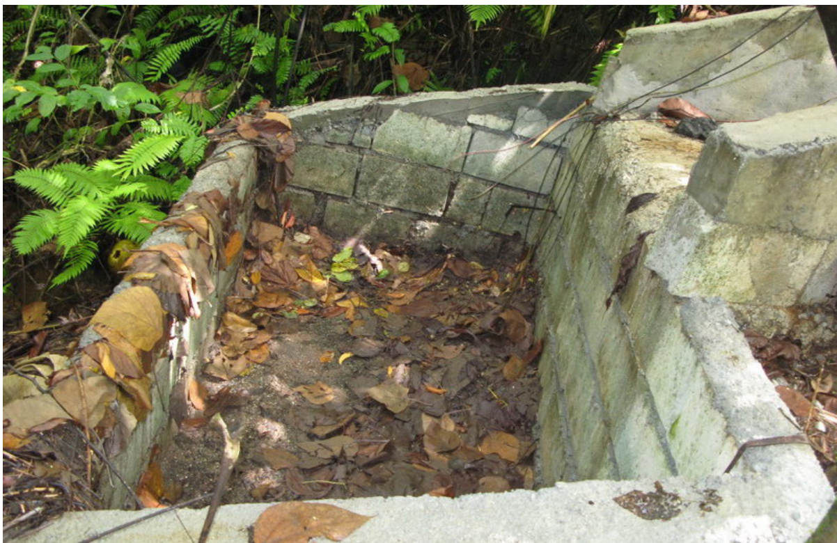
Figure 4 IWRM modification to an existing drainage ditch off the compact road in Ngerikiil aimed at reducing sediment load entering Ngerikiil River and trapping debris from road runoff
