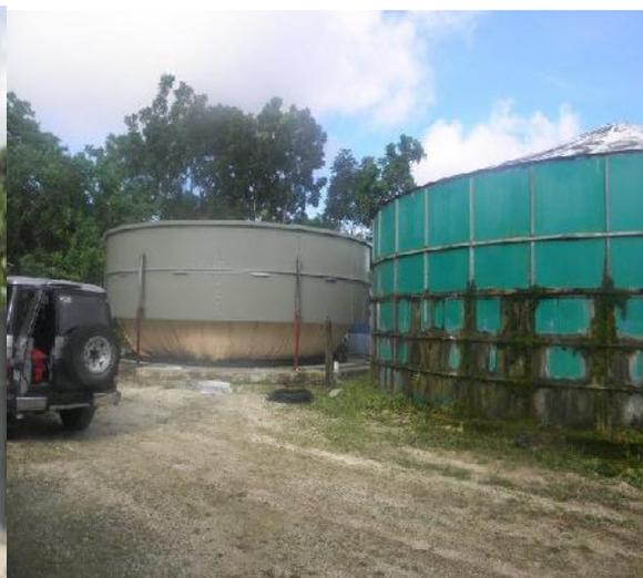
**Figure 10:** New storage (left) and old leaking storage (right)
